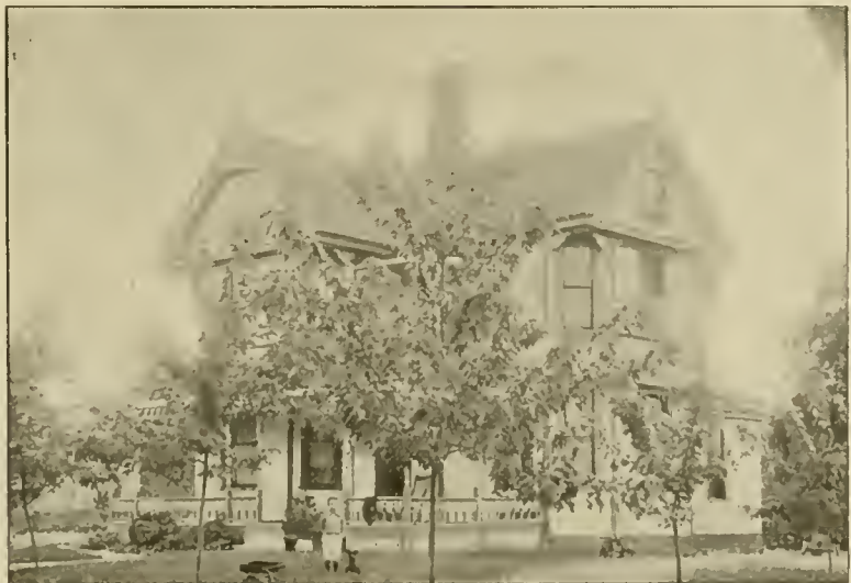
RESIDENCE OF J. M. ALBERT, on First St.
